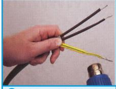
10 Apply heat and shrink the tubes. Ensure that the black tubes shrink fully.
