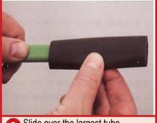
Slide over the largest tube. 8 Position the tube so it covers the end and the outside cable jacket.
