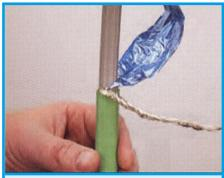
5 Pigtail the earth braid. If the cable has an aluminium sheath, remove it.
